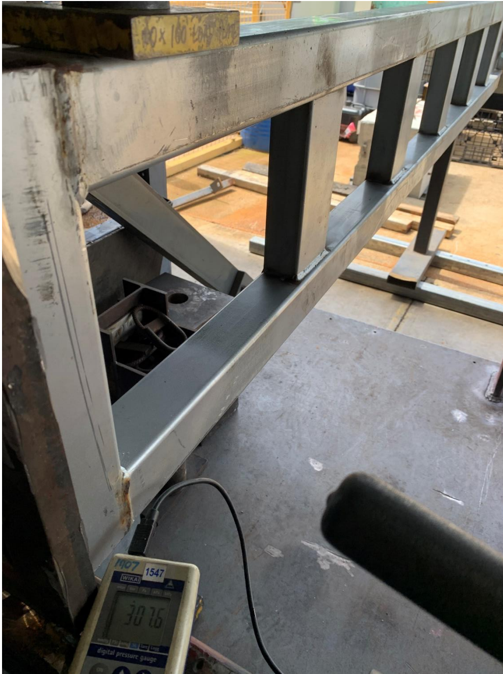
Photograph 1. General View of Lateral Static Load Testing (typical).
